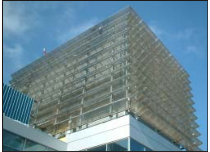
The utility plant is ringed with 640 custom-fabricated louvers.
