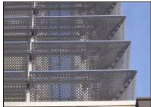
The utility plant is ringed with 640 custom-fabricated louvers.
